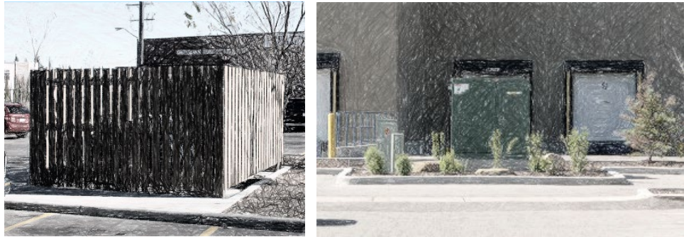
Figure 77.3.1: examples of bin and utility box screening as per 77.3(a)(b) of this section.
